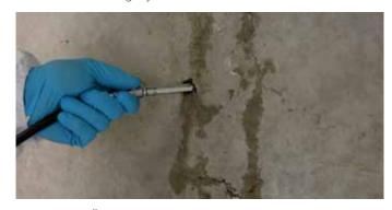
4 Inject KÖSTER IN 8 into the crack proceeding from bottom to top.
