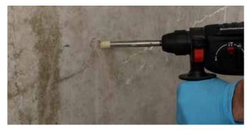
1 Drill holes along the course of the crack on alternate sides at a distance of approx. 10-15 cm and at an angle of approx. 45° towards the crack
