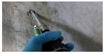
2 Install KÖSTER Superpackers in every second or third borehole. The unclosed boreholes allow pressure release during injection.
