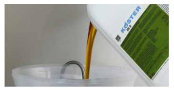
3 KÖSTER IN 8 is poured directly into the hopper of the injection pump. No mixing necessary.
