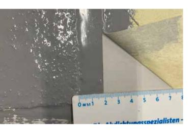
At the edge, the waterproofing must completely cover the fleece and protrude by a minimum of 2 cm.
