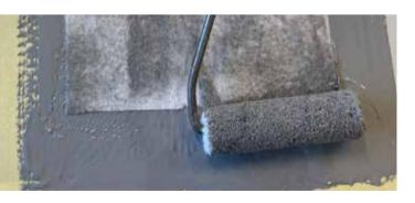
Immediately lay KÖSTER Superfleece into the fresh MS-Flexfolie without creating any creases or bubbles and press it down with a roller.
