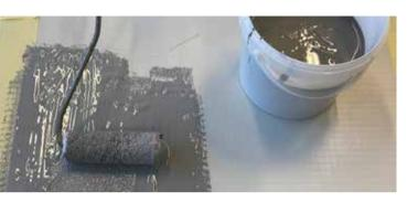
The first layer is installed with the help of a brush, roller or notched trowel.
