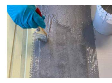
The second layer is then applied "fresh in fresh". A total layer thickness of at least 2,1 mm including the reinforcement layer must be achieved.
