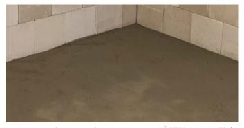
KÖSTER Mortar Tight Cement Sand Water 100 kg 10 kg Screed 25 kg 1.0 kg Sieve sizes: grain size up to 4.0 mm
