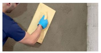
KÖSTER Mortar Tight Cement Sand Water Render 25 kg 50 kg 10 kg 1.0 kg Sieve sizes: grain size 0.2 to 2.0 mm
