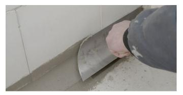
Install a round fillet on internal wall-floor junctions made from e.g. KÖSTER Repair Mortar Plus.
