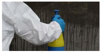
Prime the surface with KÖSTER Polysil TG 500 on salt-burned substrates.
